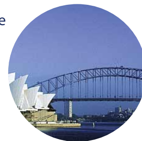
36 • Sydney Harbour Bridge
